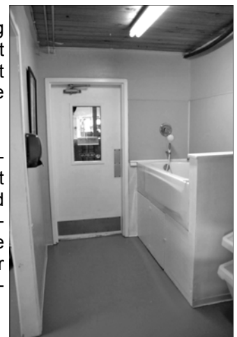
Tub room with door leading to laundry and isolation rooms.
