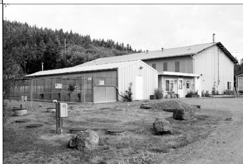
View of shelter from south east direction.
