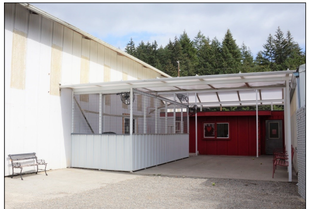
Dog yard with catio and covered roof
