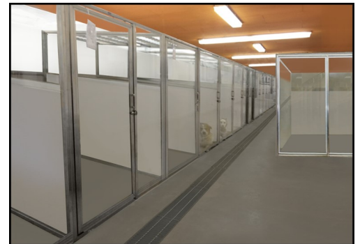
Installation of new kennels underway.
